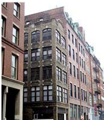
Toxic particles leaked out during renovations at 165 Friend St. in Boston (building at center).
